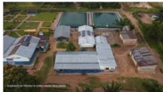
Installations de Cibombo
